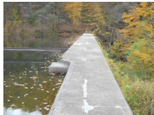
Lower Mine Hill Reservoir Dam - Concrete Repairs to Top of Dam
