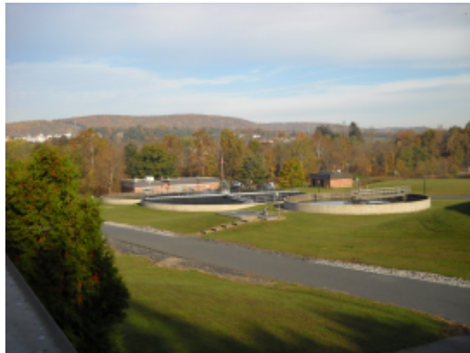
Water Pollution Control Plant Site
