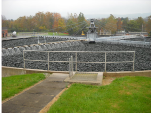
Trickling Filter
