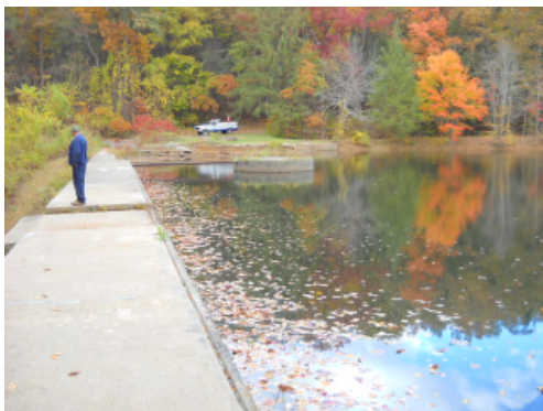
Lower Mine Hill Reservoir Dam
