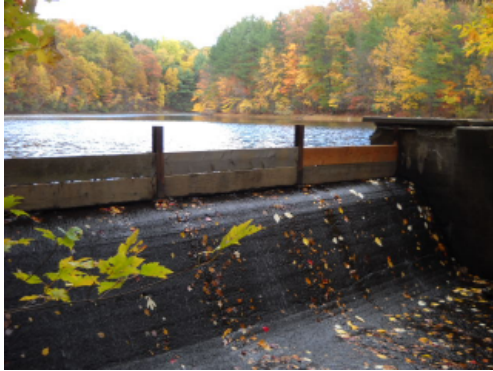
Upper Mine Hill Reservoir Dam
