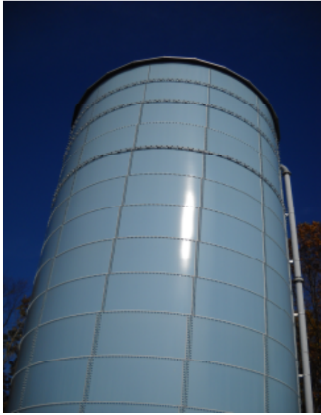
Mount Olive Township Water Storage Tank
